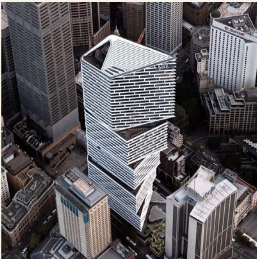
Quay Quarter Tower in Sydney's CBD doubled the size of a 46 year old building and saved 12,000 tons of embodied carbon. All credits to photographer
